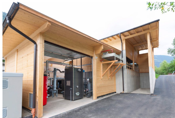
Figure 2: Wood energy gasifier systems offer an alternative to disposing of waste wood, and are common in mountain towns throughout Europe. Pictured is a 135kW biomass gasifier system in the South Tyrol region of Italy, near the Dolomites.
